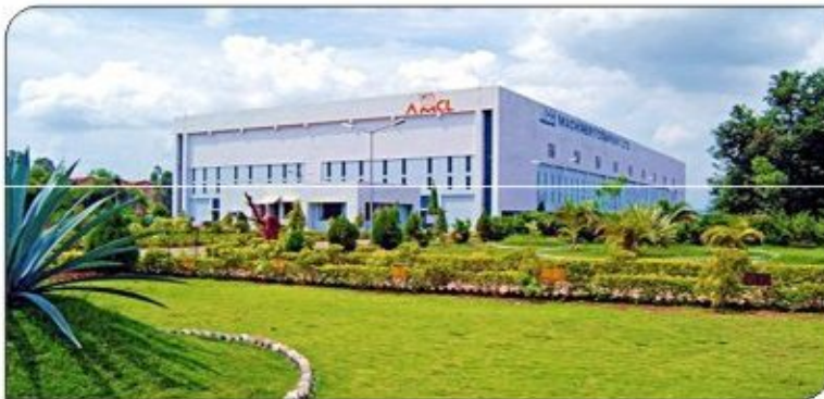
Works at Nagpur
